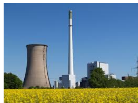
Figure 2.3: An example Coal Power Plant
