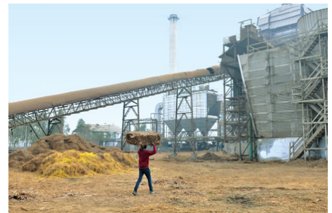
Figure 20.3: A rice straw power plant, India
