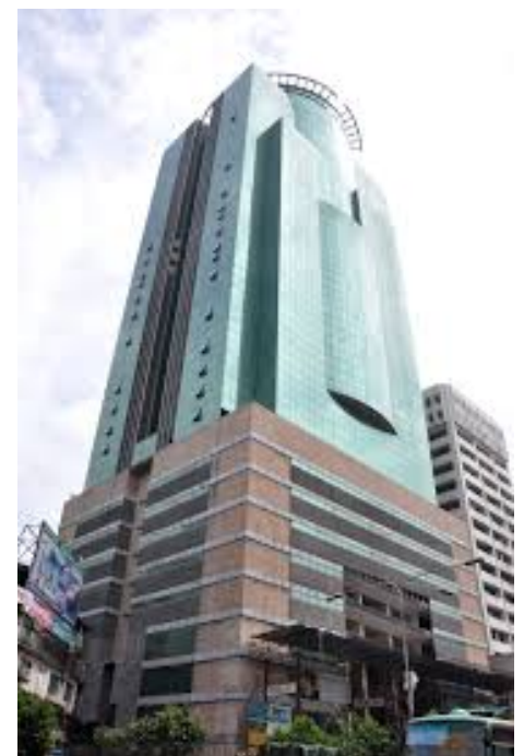
Figure 35.3: A commercial office building, Bangladesh
