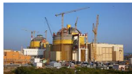
Figure 5.3: A Nuclear Power Plant under construction
